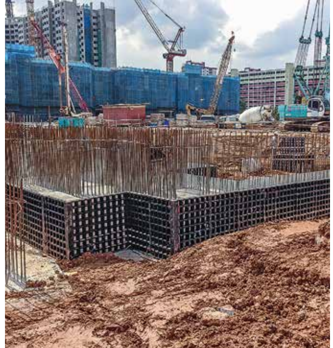
The DUO panels were ideal for forming small-scale concrete components with low surface requirements.
